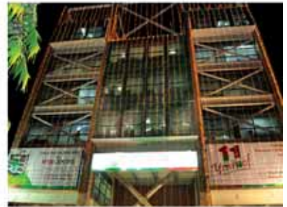
'MTB Centre' sets a milestone in green and energy consciousness in the corporate world of Bangladesh. The building is an intelligent building as it has adaptive technology in energy consumption and environment-saving, which is located at 26, Gulshan Avenue, Dhaka 1212. 'MTB Centre' was embellished with lights and colors on October 24, 2010 on the 11th Anniversary of the bank.
